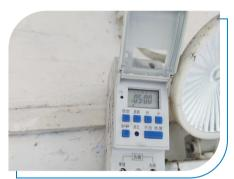
Installation of time control switches on the laboratory lighting for improvement
